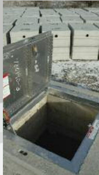
Commercial Lift Station Riser (foreground), Septic Tanks (background)
